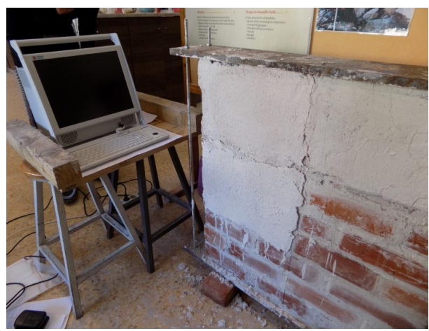
Application of the renders on the masonry sample.
